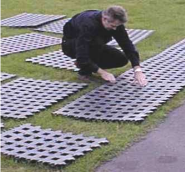
Sections arranged on the ground
